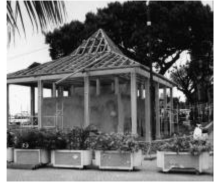
visitor center combining concrete, steel and wood construction
