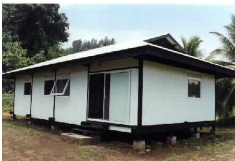
A new home built to the government standards of French Polynesia; framed with U.S. Douglas fir
